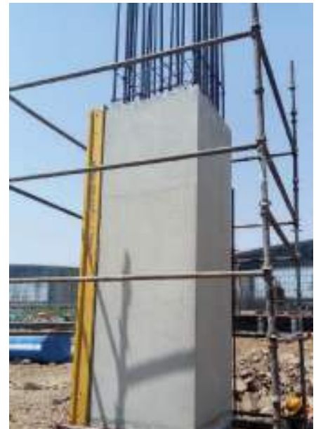
Form Finish Column Concrete using GGBS upto 50%
